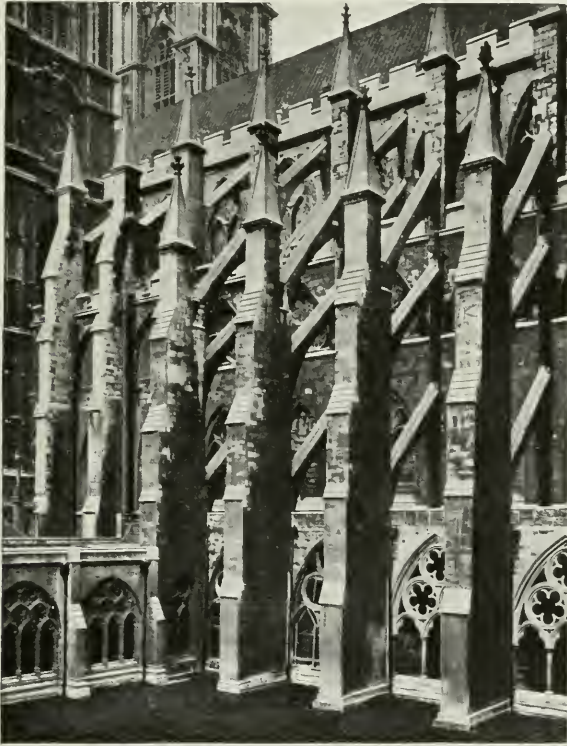
34. Buttresses to Nave, Westminster Abbey.
